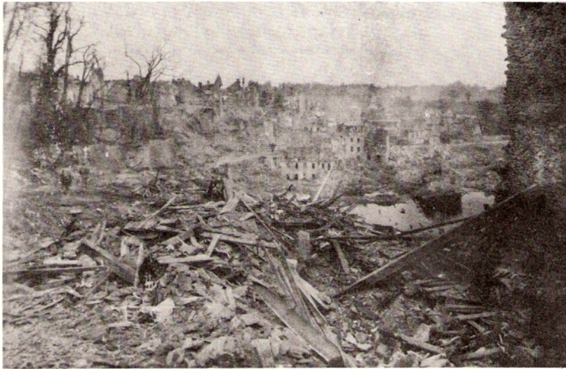
STREET SCENE, NORTH ST. LO, BEFORE BEING CLEARED
