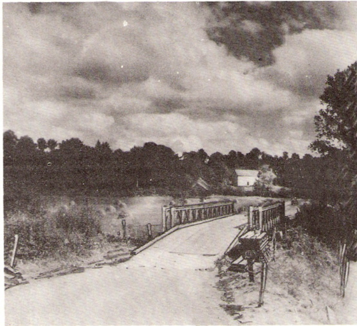
"C" COMPANY'S BAILEY BRIDGE AT GER, FRANCE. AUGUST 1944
