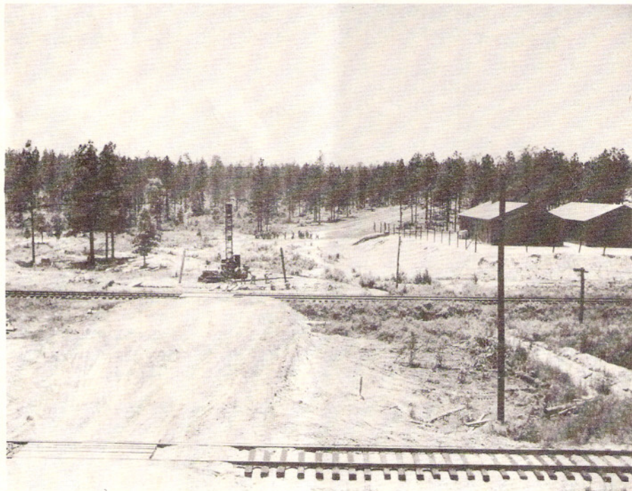
THE ROAD CONSTRUCTION PROJECT CAMP SHELBY, MISSISSIPPI
